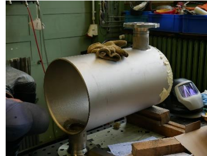
Outer vessel welding
