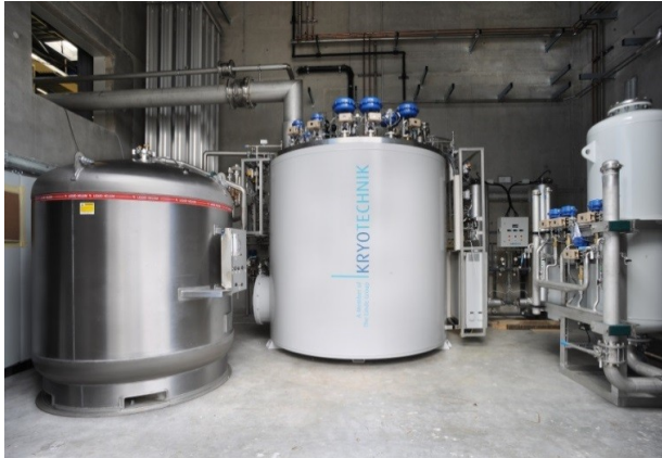
Coldbox in the cryo room (1.5 kW@4.5K eq.)
