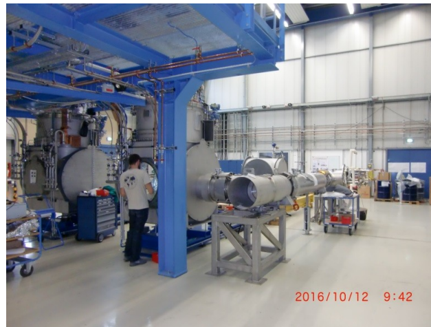
Jumper-line during installation on the side of one Feedbox
