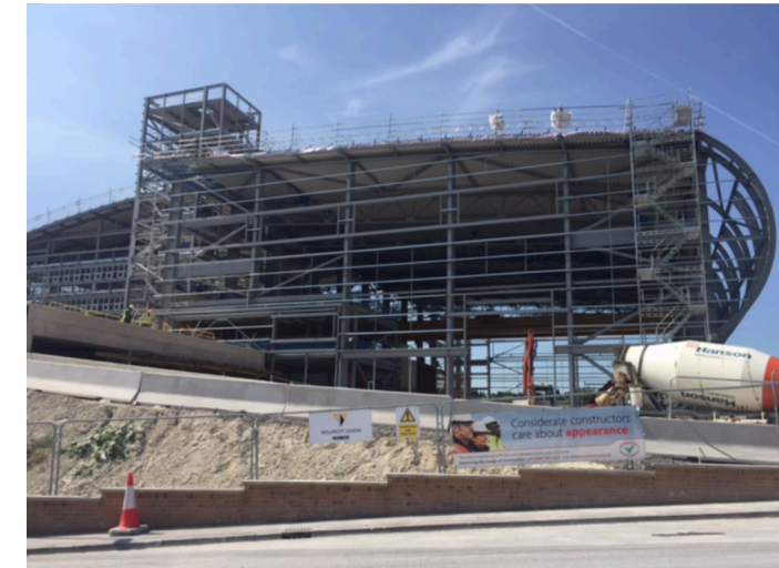
Construction of R106 where STFC will pre-build LOKI and FRIEA
