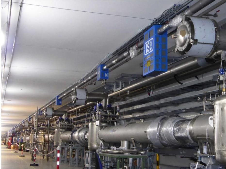
Distribution of 2 frequencies (352.21 MHz and 704.42 MHz) from MO to the tunnel
