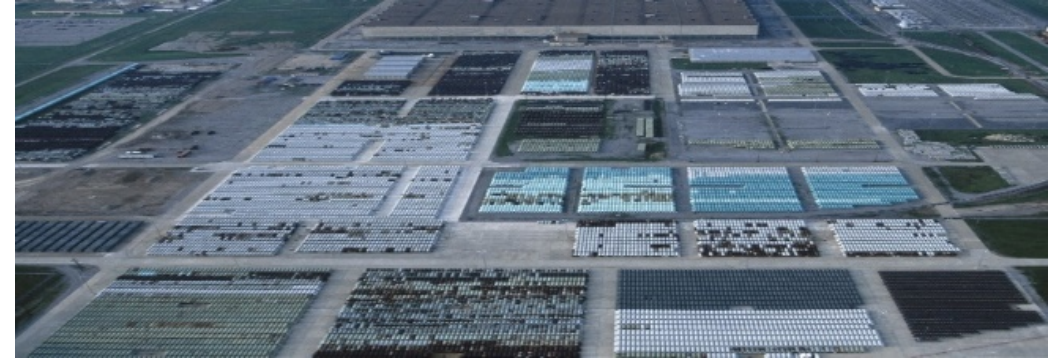
DU storage facility in Paducah, KY
