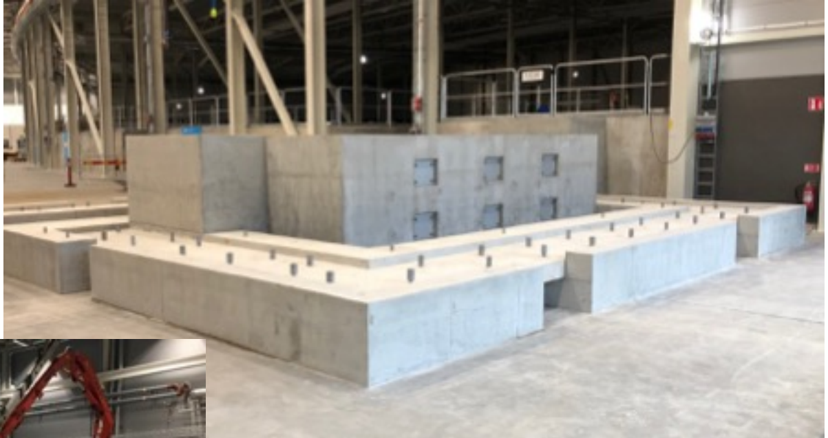
January/February: Internal cave floor cast-in-place
