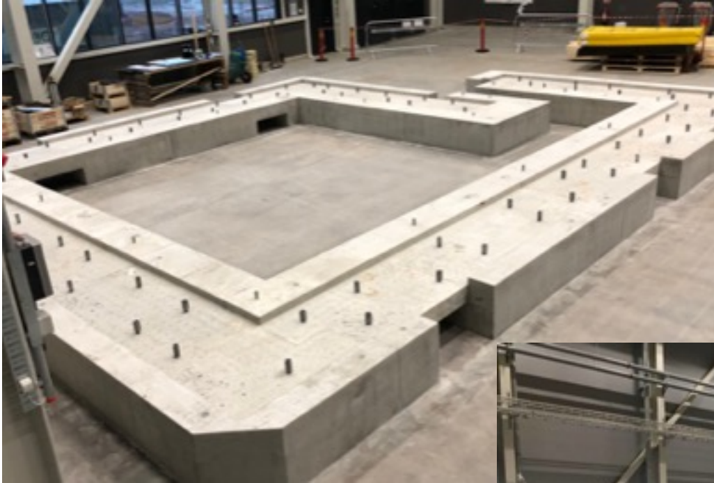
Foundation cast in place December 2019
