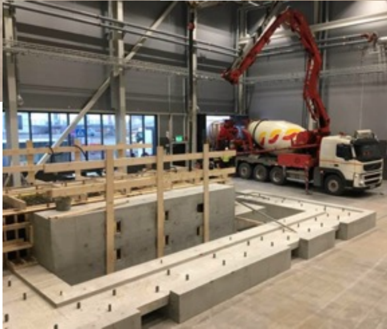
January/February: Internal cave floor cast-in-place
