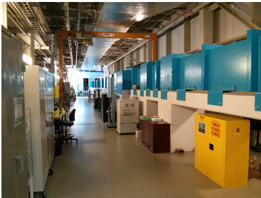
Figure 2: BASIS beamline at SNS, out of line of sight of the source. The shielding is relatively light, and the guides are supported on a raised concrete platform.
