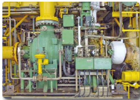
Turbo expander installation. Over 600 O&G units in the field
