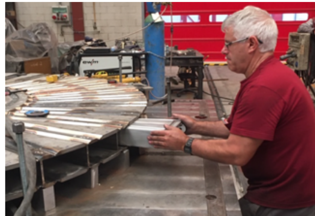
Target wheel ribs in place and tack welded. Tested with dummy cassette
