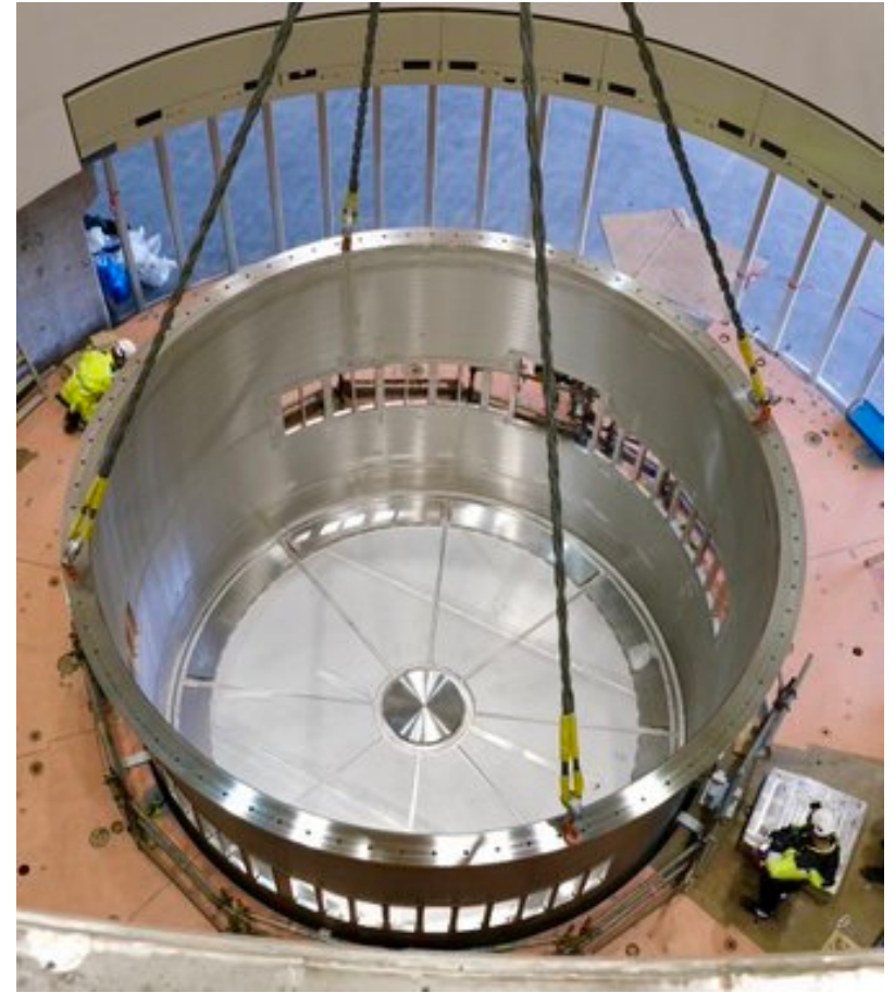
Monolith Vessel Arrived in Lund, lower half now installed
