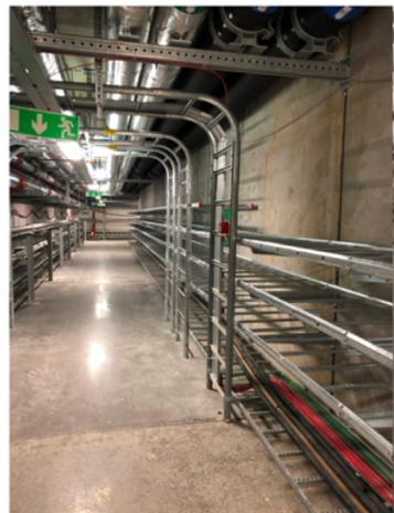
Electrical infrastructure (cable trays / raceways) in D-building galleries
