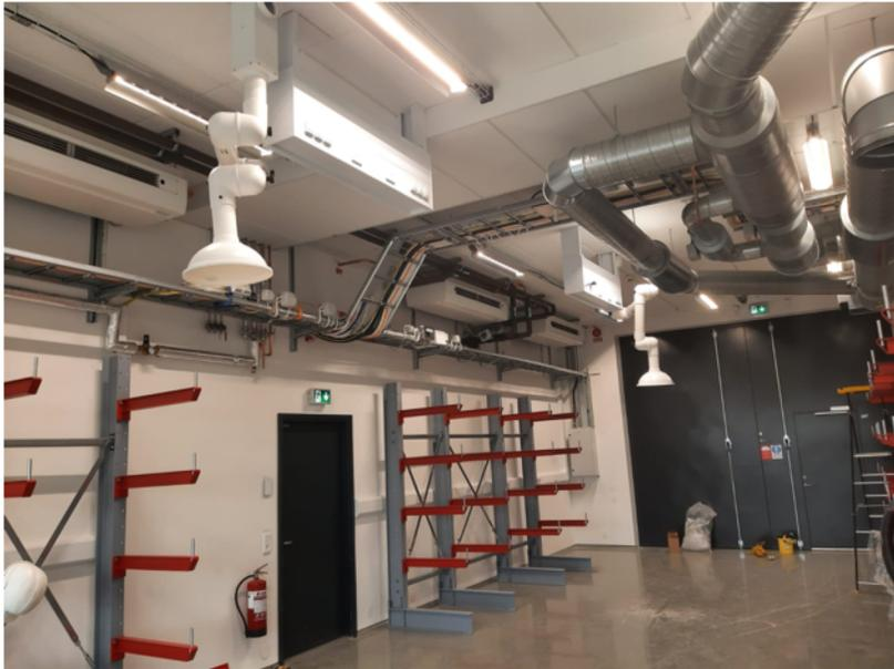
Shelves and fume extraction points installed in E04 Detector area
