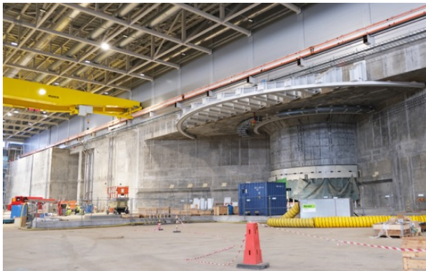
D01 crane consoles welded in place; D02 Transport Hall entrance gates; E02 part 2 installations.
