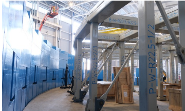
Bunker Pillar system installing in D03, outer west wall shielding 95% assembled.
