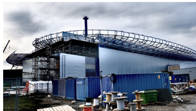
Structural steel and cantilever roof takes shape as well as final building cladding
