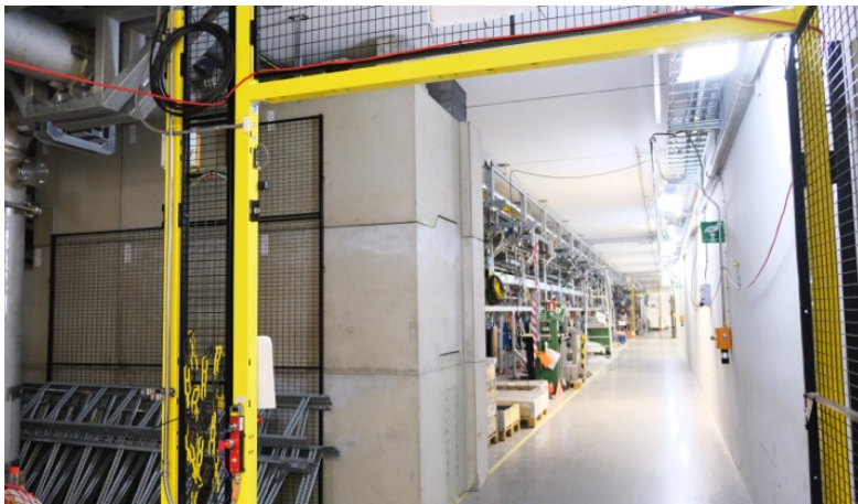
Temporary shielding wall.
