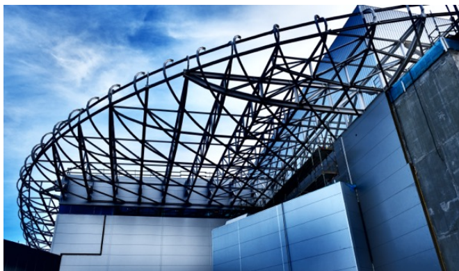
Structural steel and cantilever roof takes shape as well as final building cladding
