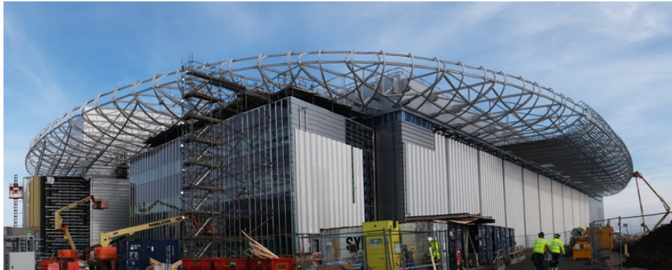
Structural steel and cantilever roof takes shape as well as final building cladding
