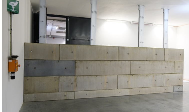
NCL Shielding: front end penetrations, front end chicane wall and drop hatch shielding.
