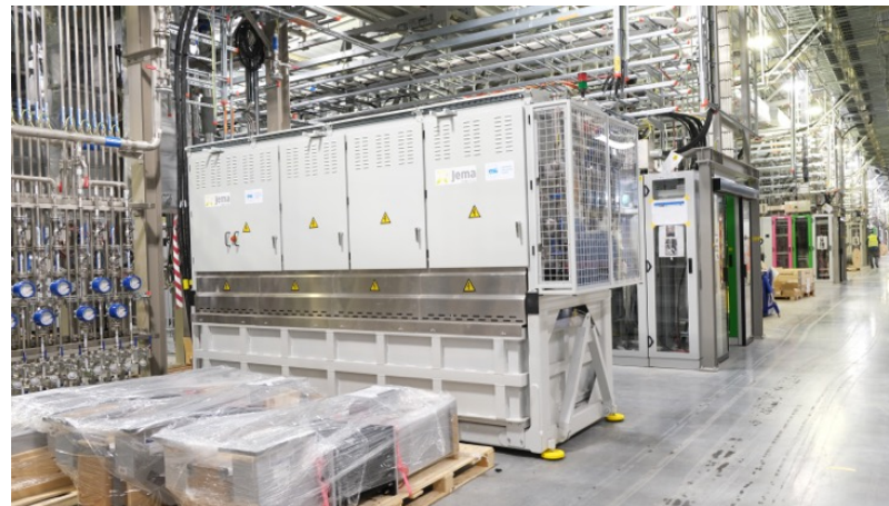
NCL Modulator #1 and Klystron operated at full power, 5 of 6 NCL Klystrons in place.
