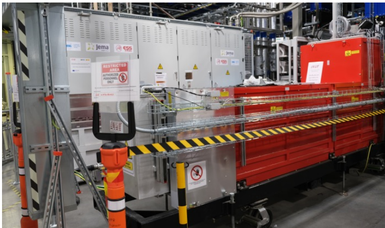
NCL Modulator #1 and Klystron operated at full power, 5 of 6 NCL Klystrons in place.
