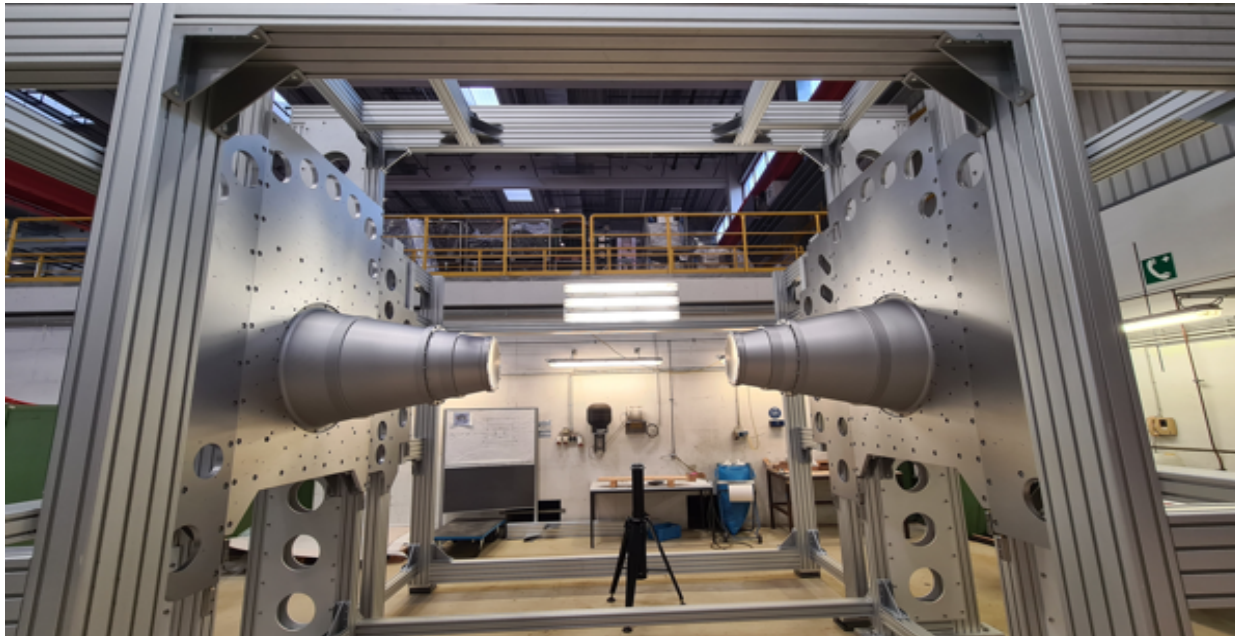
End-cap det. plates & vacuum cones are installed, Jan. 2021
