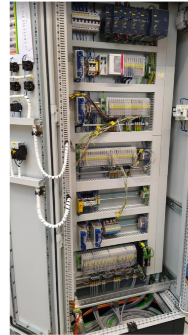
Motion Control cabinet for Estia at PSI
