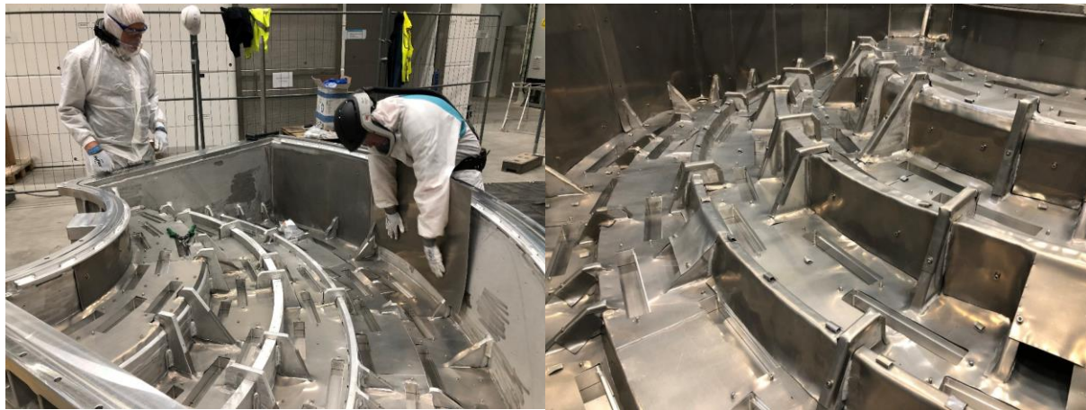
Figure 3:(Left) Two safe technicians mounting cadmium plates. (Right) Cadmium covered on the spectrometer tank floor
