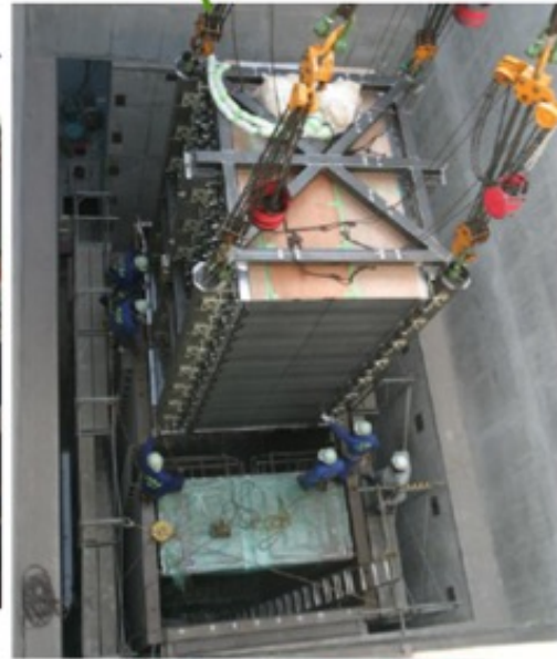
Beam Dump (water cooling)
