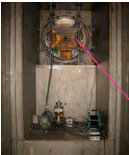
Temporary seal on the target trolley insertion port of He-vessel
