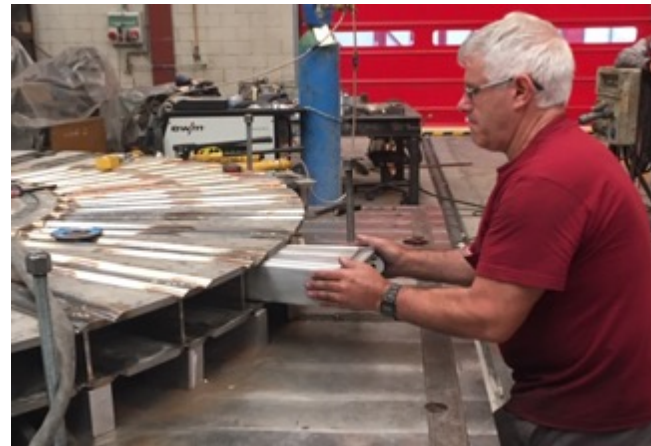
Target wheel ribs in place and finished welding.
