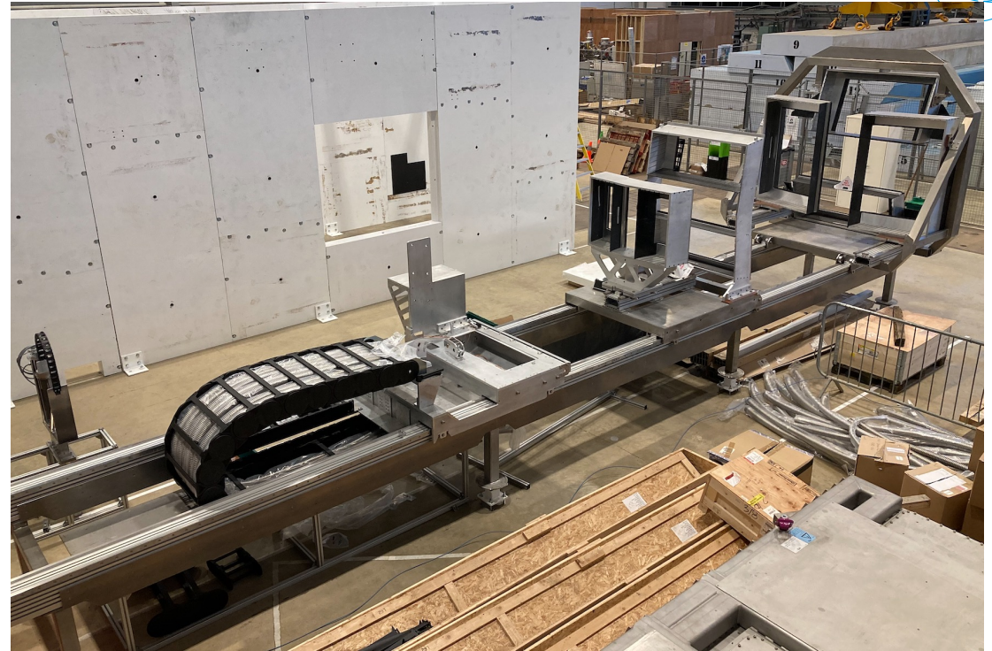
Detector mechanics prebuild at ISIS
