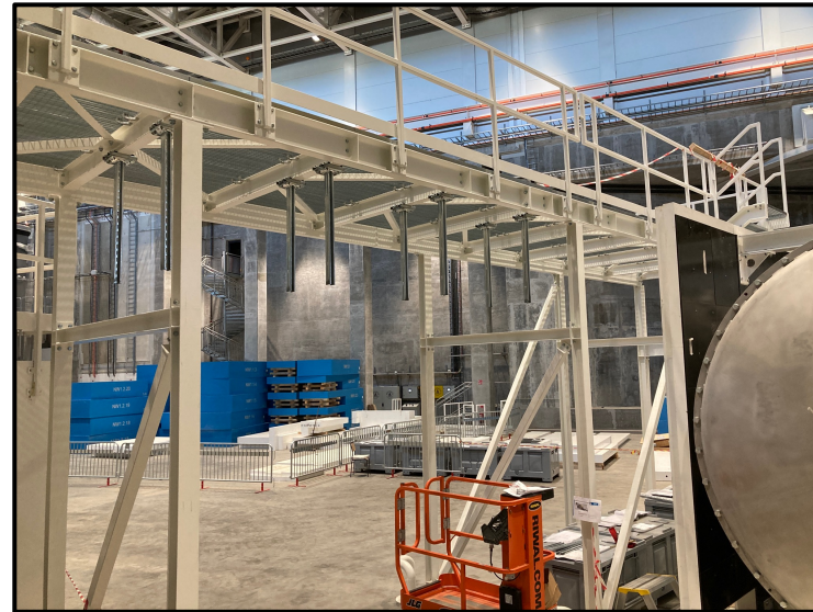
Raceways and other infrastructure for electrical and detector cabling
