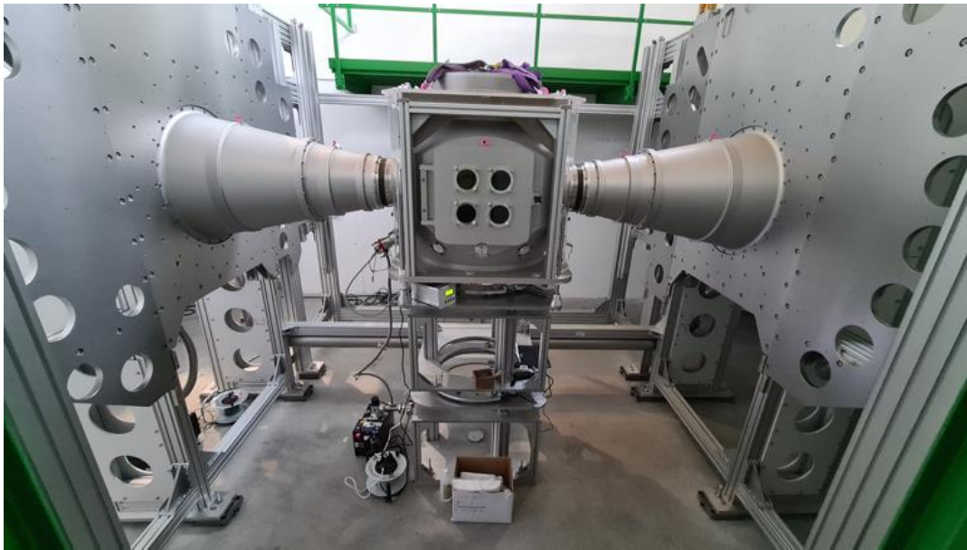
Figure 3 Sample vessel installed on sample vessel support inside detector support structure in the DREAM cave.
