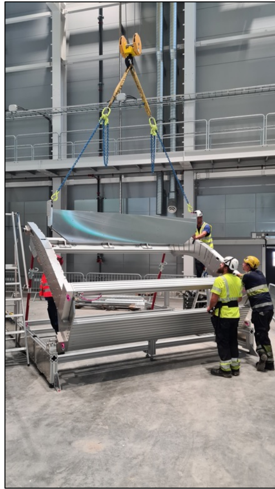
Loading mantle "detectors" with hall crane
