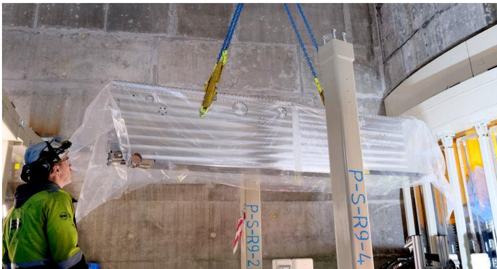
Figure 1 DREAM NBOA is being installed.
