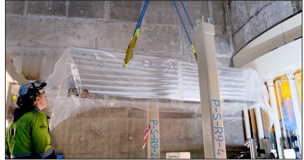
DREAM NBOA is being installed
