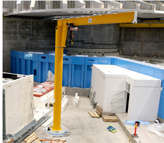
LoKI crane and TBL cave
