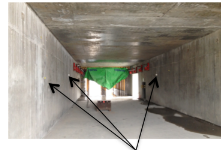
Tunnel network references already installed.
