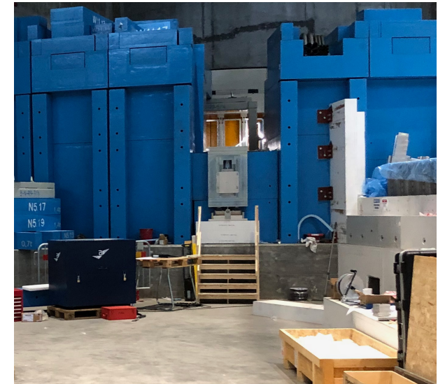
Freia feedthrough installation
