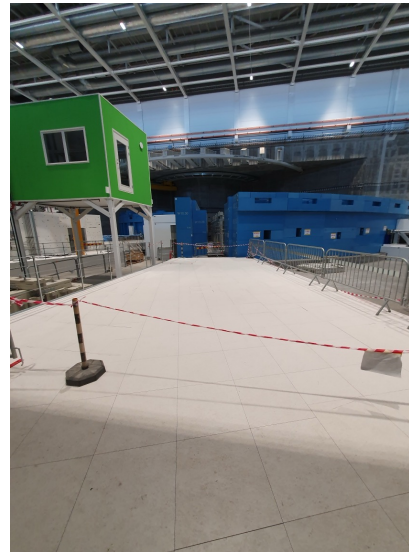
NW raised floor
