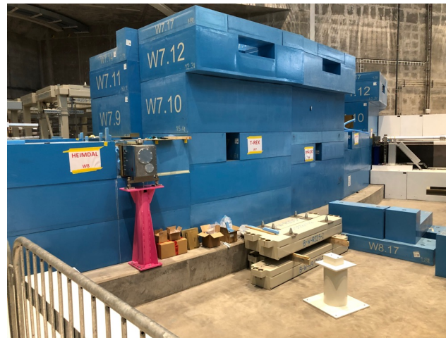
Heimdal Feedthrough installation
