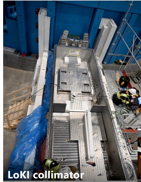
LoKI positioning the collimation blocks inside the vacuum vessel
