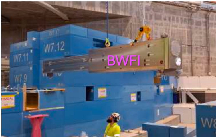
Heimdal Bunker wall Insert installation.
