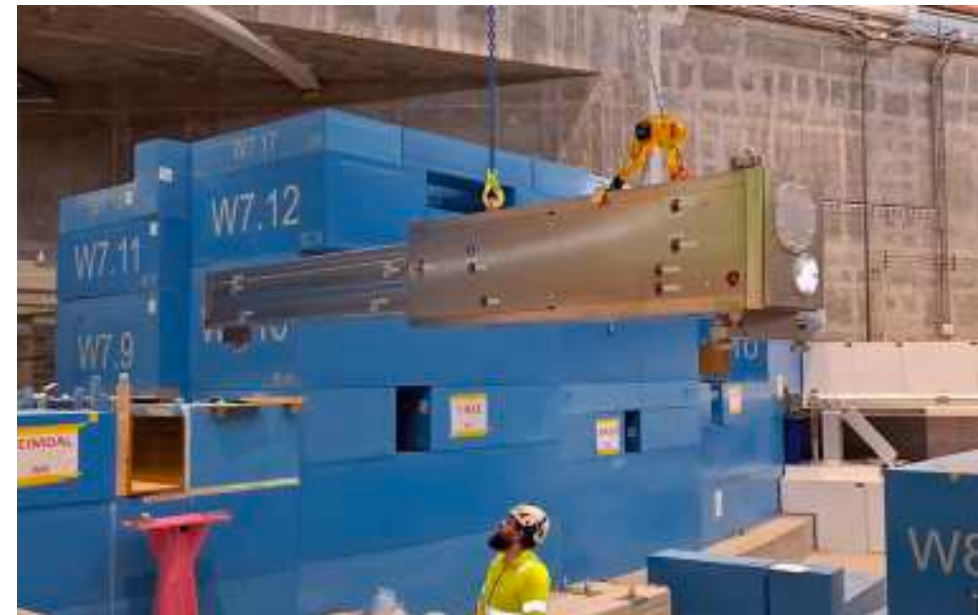
Bunker wall feedthrough insert is installed
