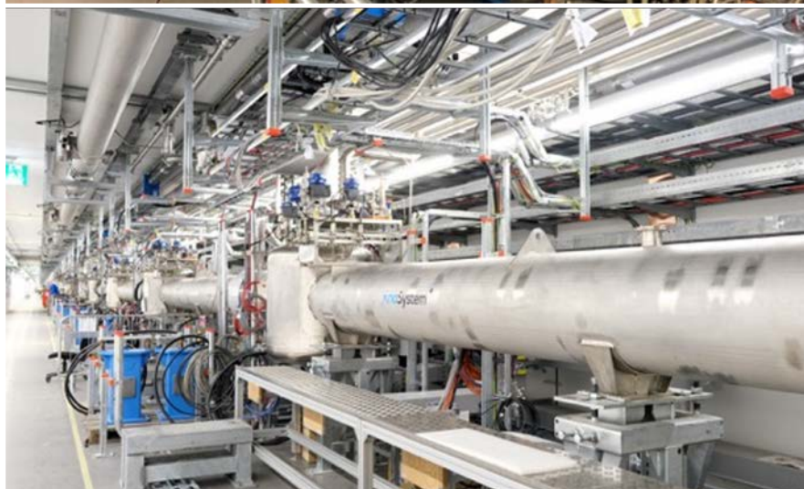
Cryo Distribution Line Testing underway, followed by cryomodule installation
