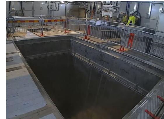
Storage Pit Lid Installation
