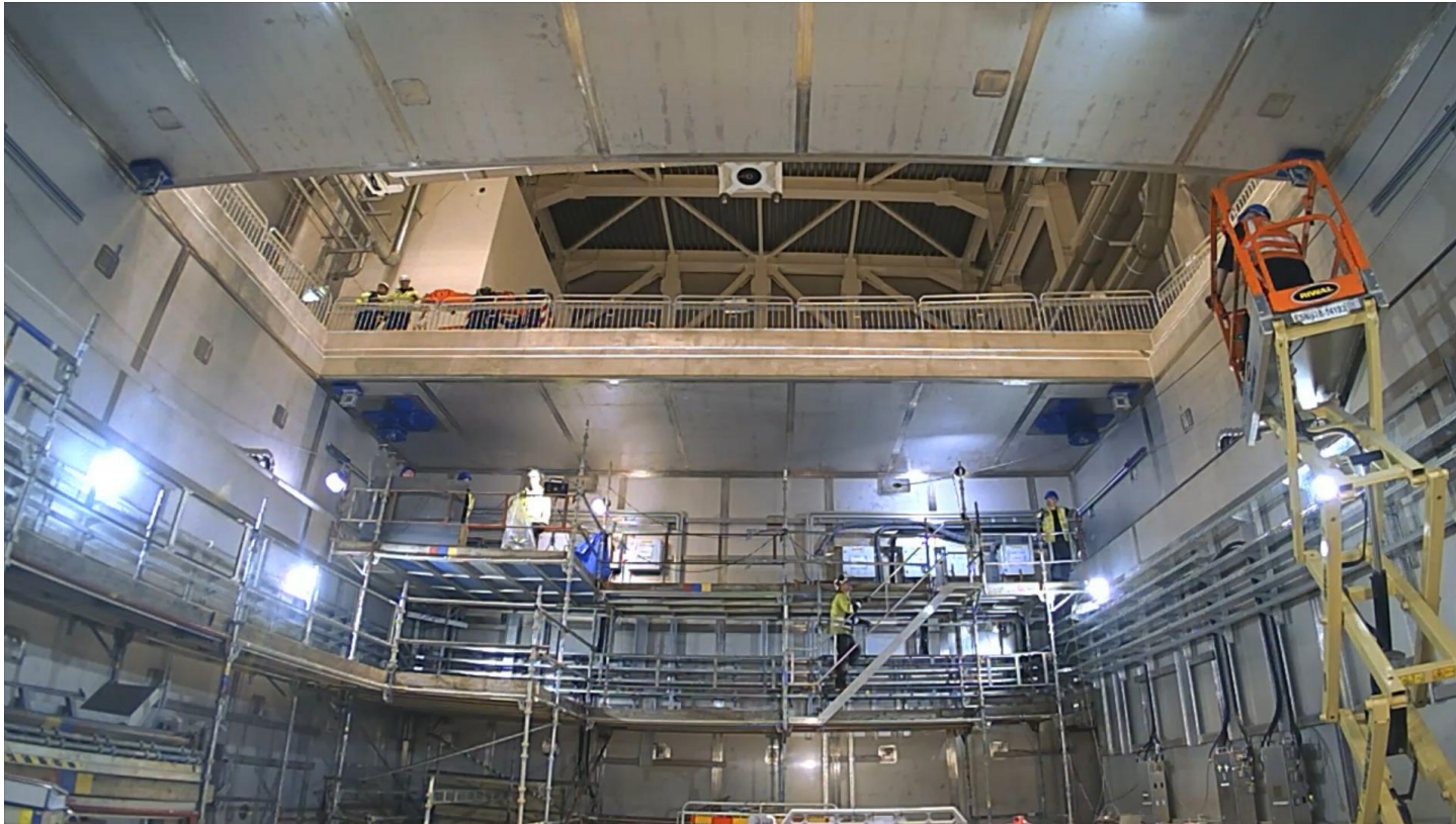
Grapple Crane Installation
