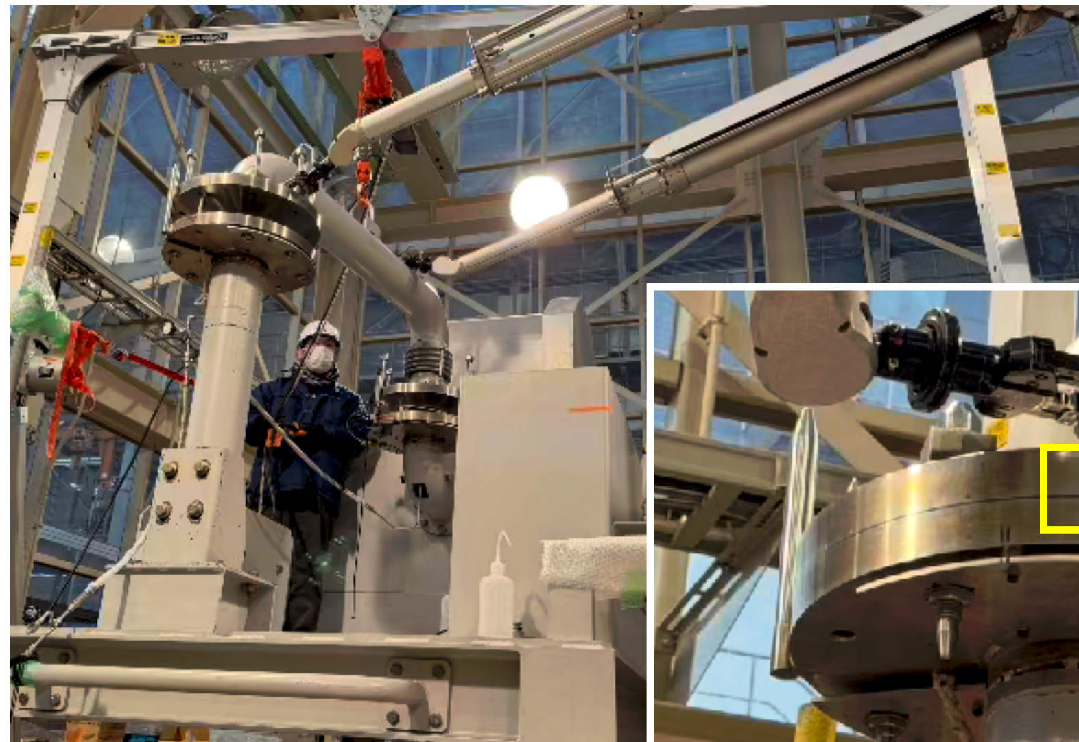
Jumper pipe setup by crane and manipulator
