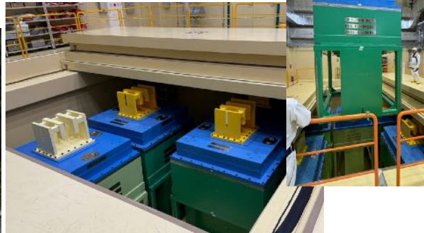
Storage pit in RAM building
