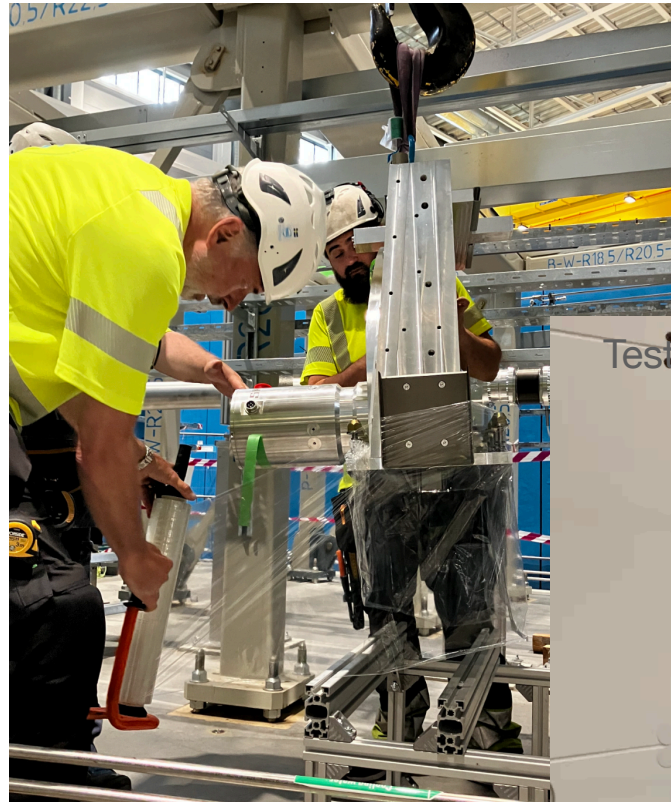
Installation of BW choppers in bunker. All choppers tested and accepted
