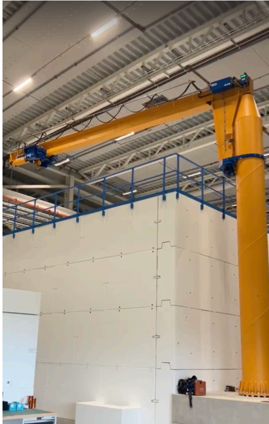
Completion of cave and crane installation
