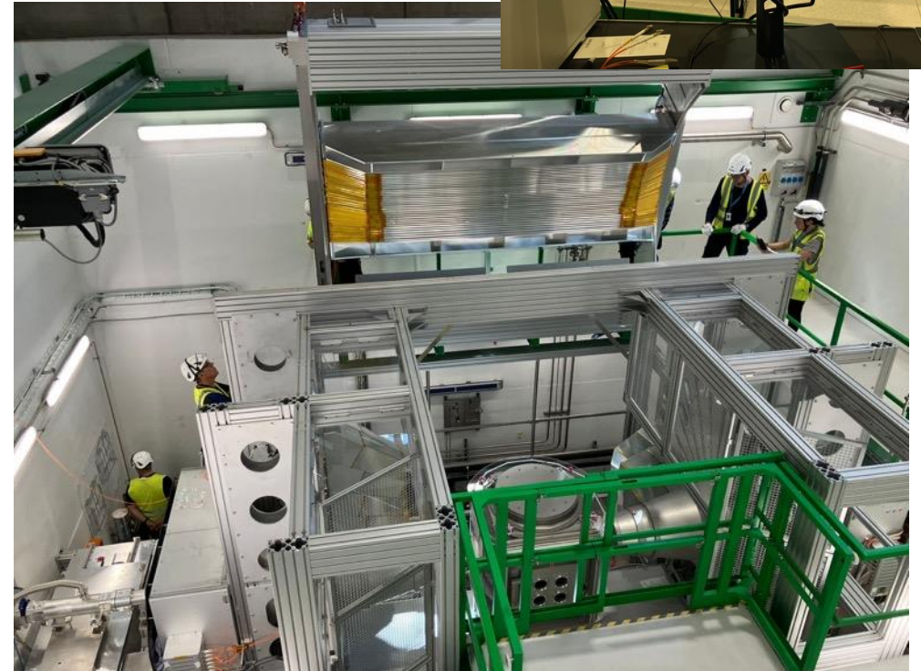
Mantle detectors installation
