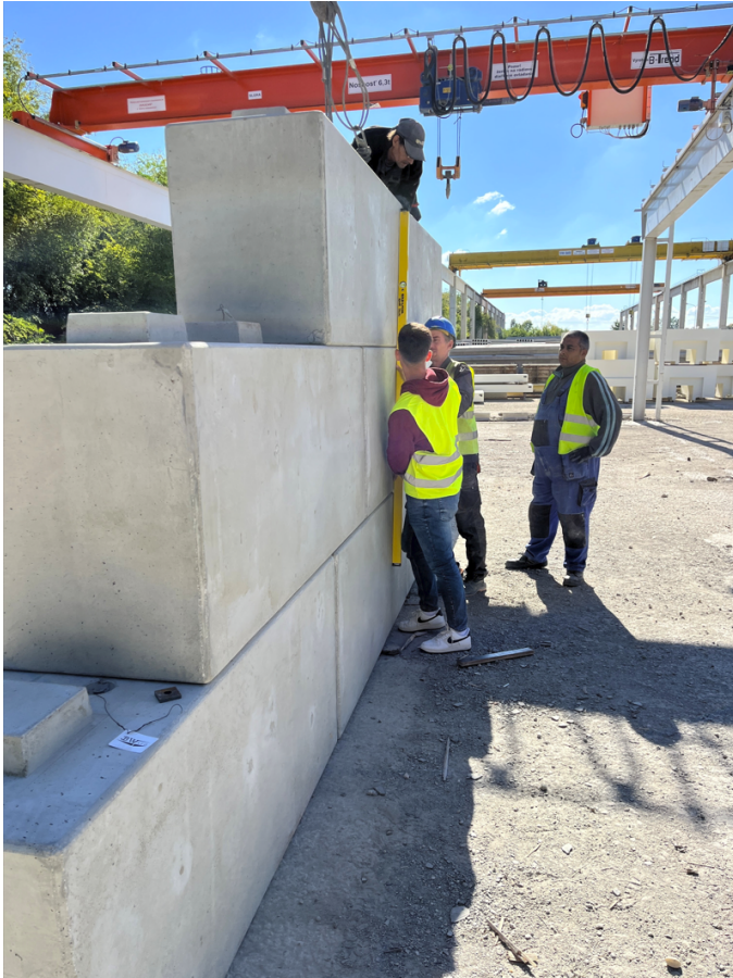
Manufacture of "Lego" concept Heimdal cave concrete blocks contractor Mirrotron.
