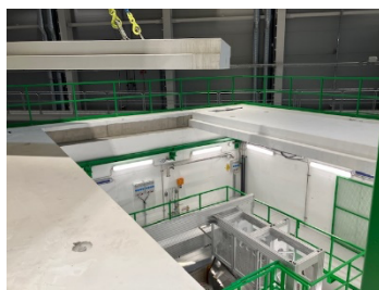
Figures 1: Craning of mantle detector to its final position – Closing of the cave roof - Ar-CO 2 gas panel for detector inside the cave.
