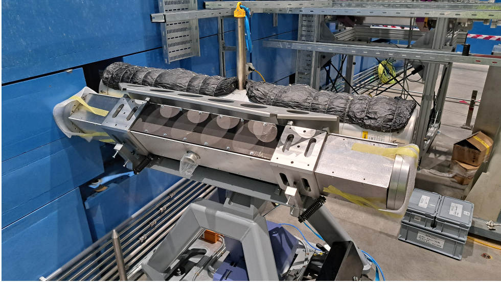
FIG. 3. The installed Heavy Shutter.
