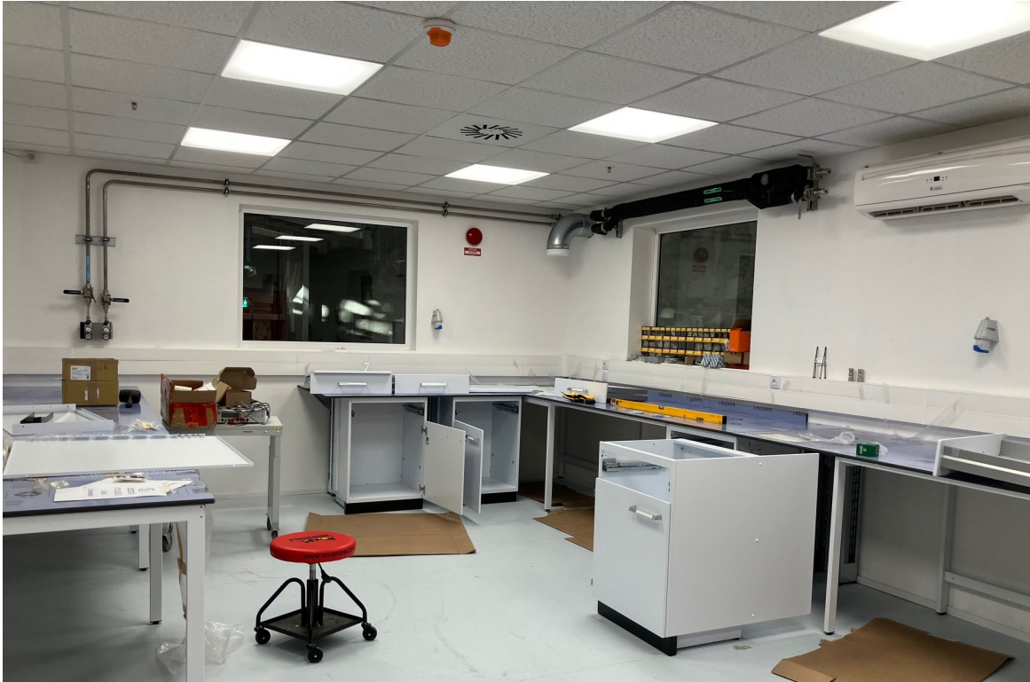
Fitout of the lab. space ongoing
