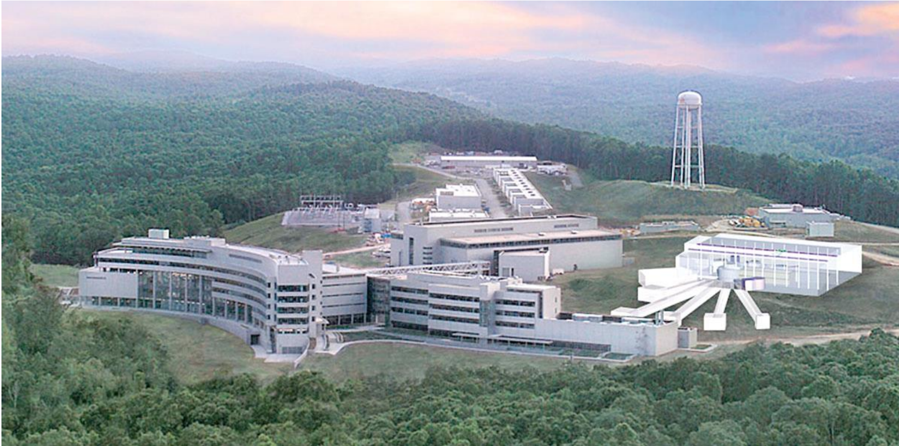
Spallation Neutron Source in Oakridge
