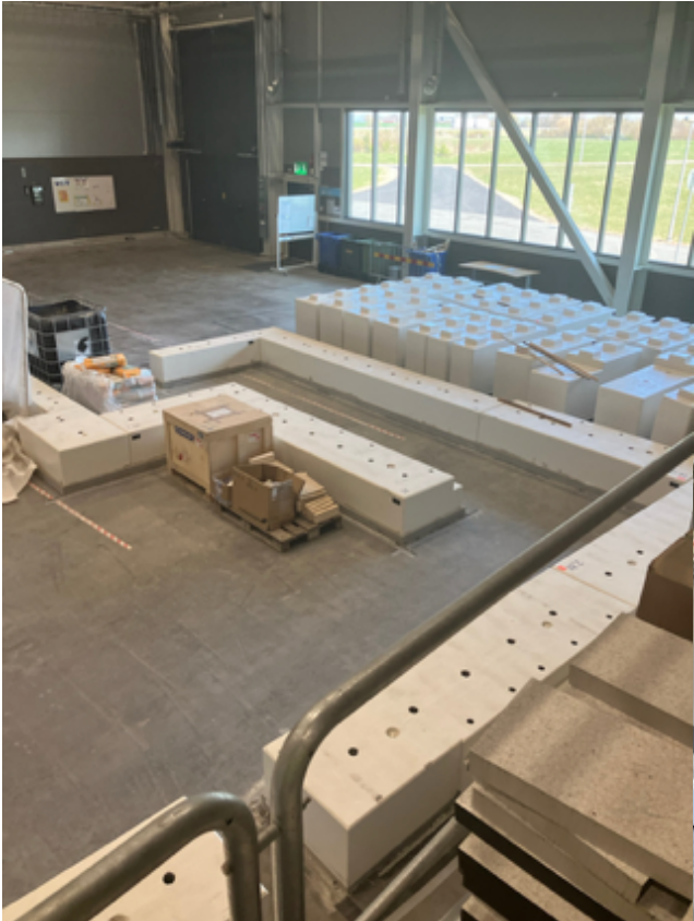
Heimdal Cave foundation installed at ESS and wall blocks delivered to be installed in April/May 2026..
