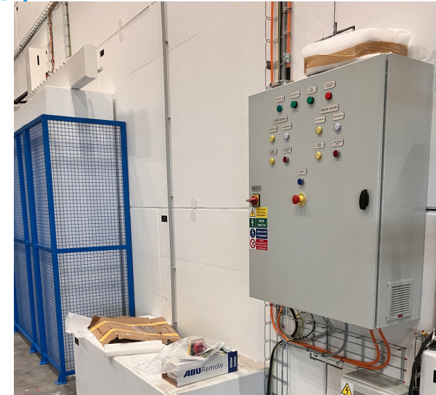
Testing of cave block door.
