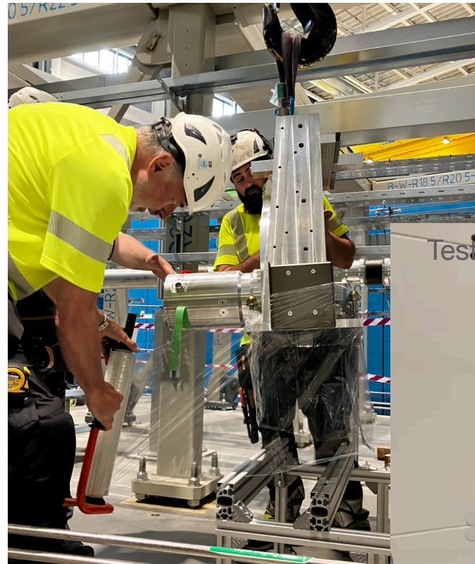
Installation of BW choppers in bunker. All choppers tested and accepted
