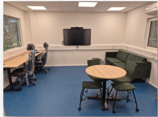
Control hutch fit-out started
