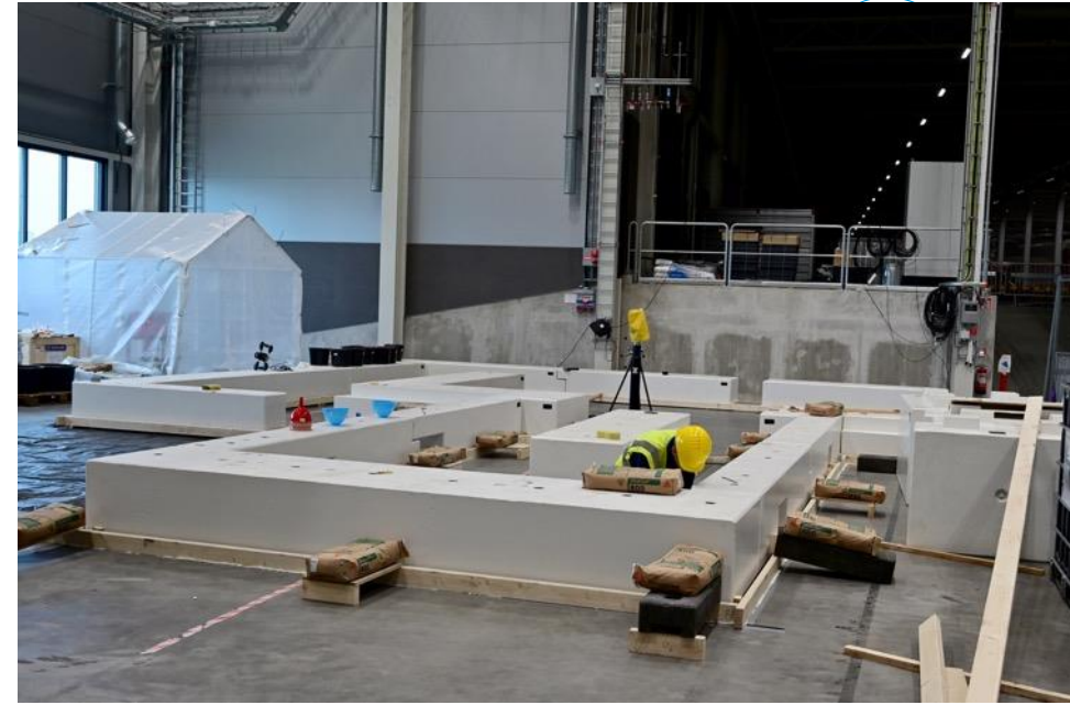
Cave slab installed
