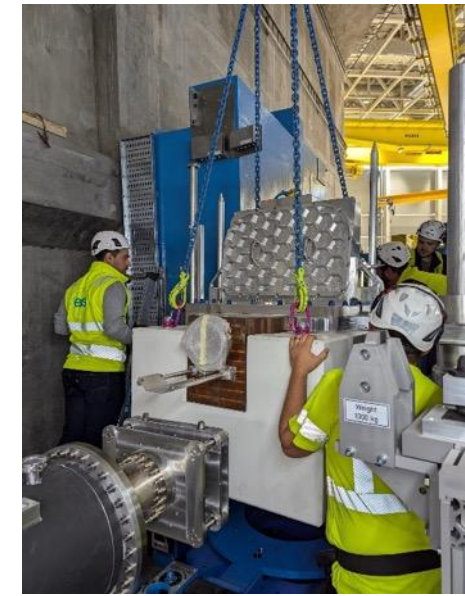
Chopper System (B4C Resin Al-disc, Diameter 700mm, 14Hz)
