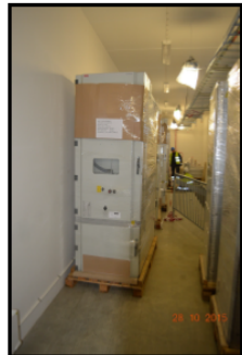
Photo 4, H05 ABB Switchgear
