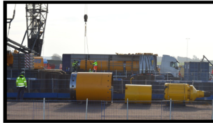
Photo 1, Drilling Equipment for Monolith Piles
