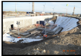
Photo 1, G01 Emergency Exit nr E31
