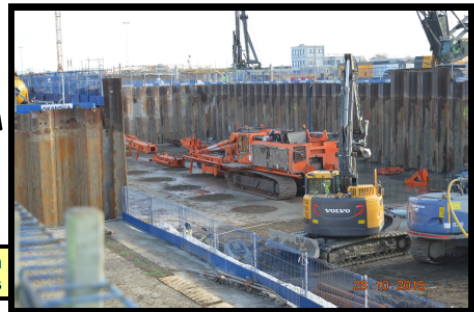
Photo 3, Rig for Monolith Piles in D02
