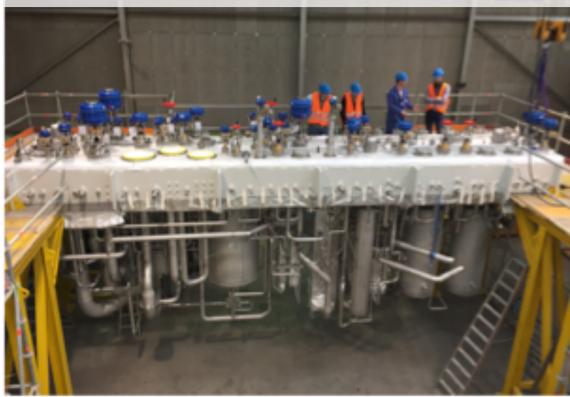
Figure 1: View of ACCP Under Final Assembly at Vendor.
