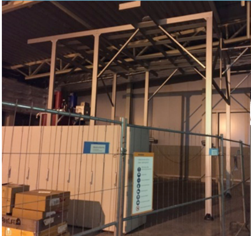
Support structure for RF Distribution System and Water Piping
