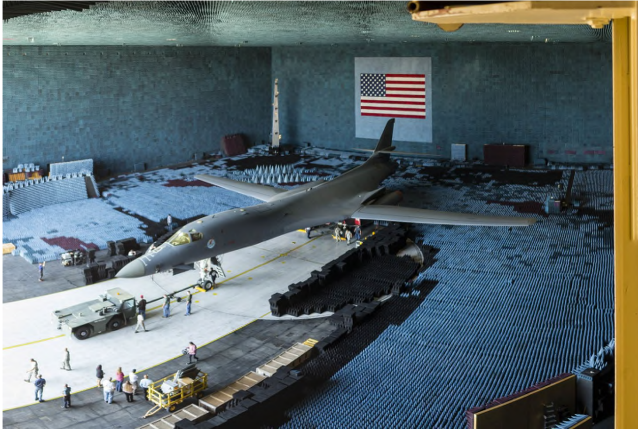
Benfield Anechoic Facility, Edwards Airbase Photo: Wikipedia, Public Domain
